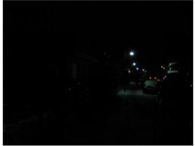
illumination with 50 watts of sodium steam lamp
